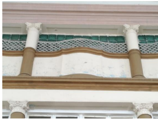
Figure C18: Galleries. Southern wall. Third floor. (Author, 2018).
