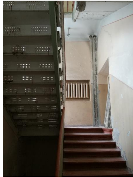
Figure 2-35: Staircase. Second half-floor (Author, 2018).
