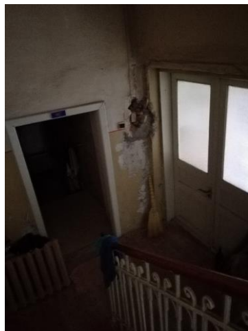
Figure 2-16: Entrance to the toilets (left) and courtyard (right). (Author, 2018).
