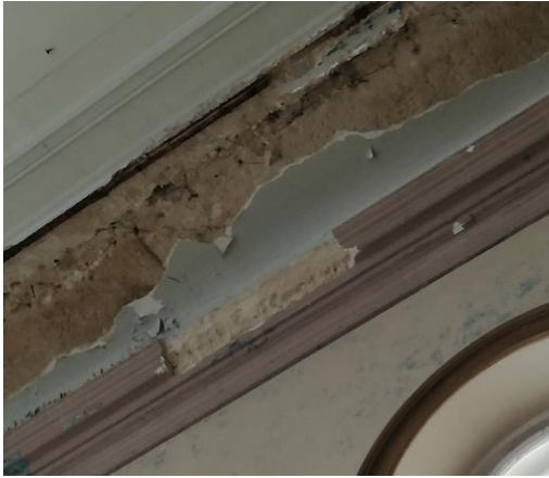
Figure C15: Prayer hall. Ceiling over the windows. Northern wall. (Author, 2018).
