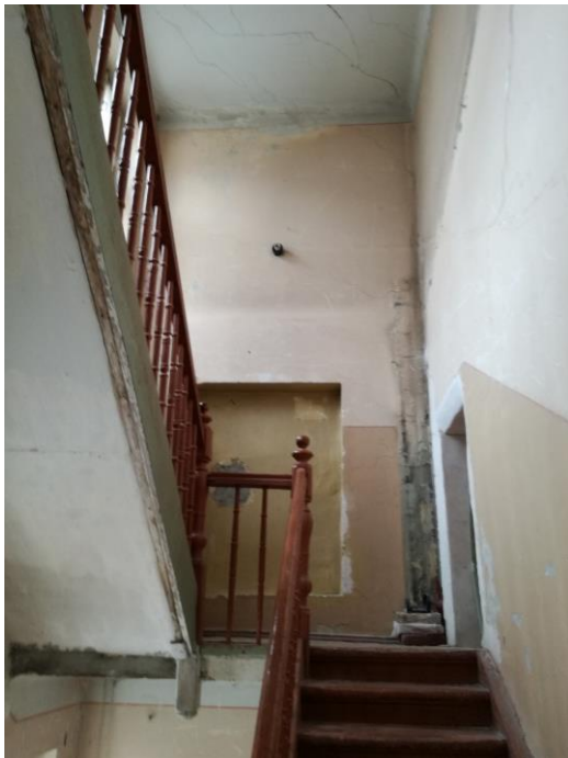
Figure 2-44. Staircase. Third half-floor. (Author, 2018).
