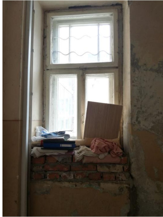
Figure C321: Staircase window. First floor. (Author, 2018).
