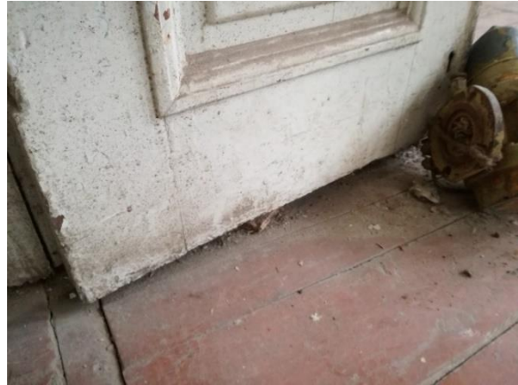
Figure C16: Trimmed door to the prayer hall. (Author, 2018).
