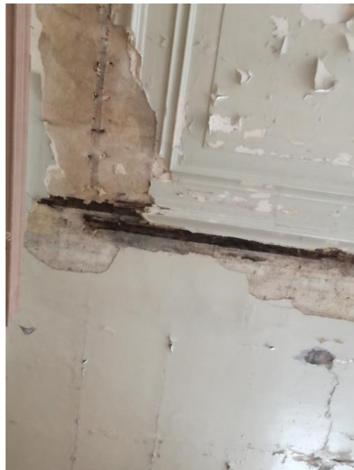
Figure C14: Prayer hall ceiling. Uncovered steel beams. (Author, 2018).
