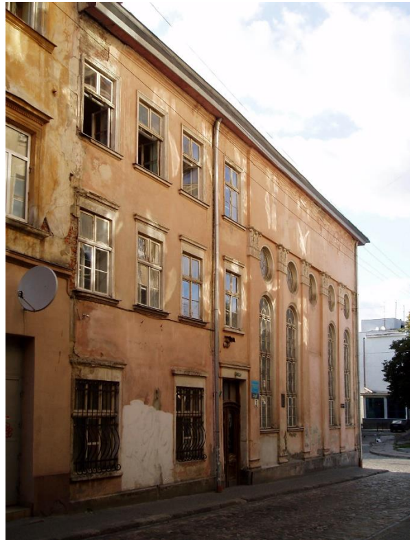
Figure 2-10: East facade. Building transition. (Nazar, 2011).
