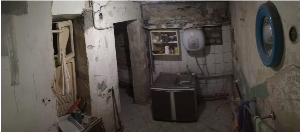
Figure 2-31: Toilets. General overview. (Nazar, 2018).
