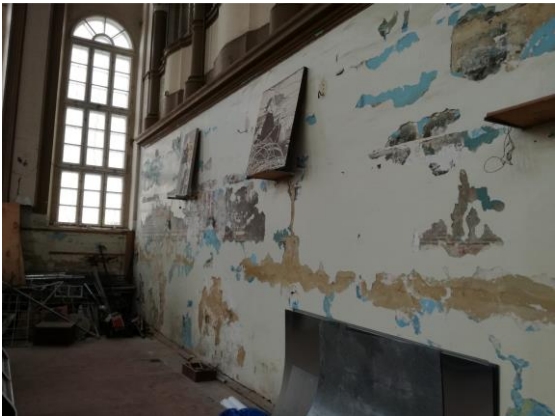
Figure 2-23: Prayer hall. Paintings on the southern wall. (Author, 2018).
