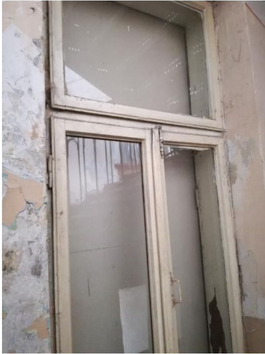
Figure C31: Staircase window. First half-floor. (Author, 2018).
