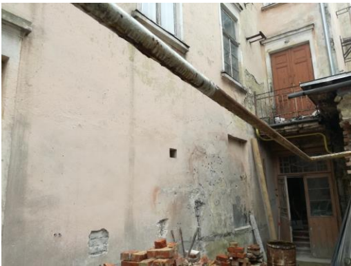
Figure C7: Western wall. Courtyard view. (Author, 2018).
