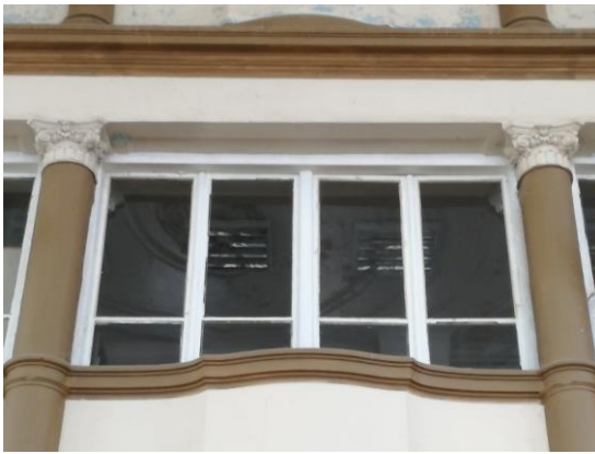
Figure C17: Galleries. Southern wall. Second floor. (Author, 2018).
