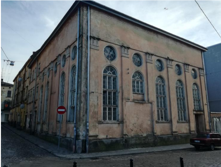
Figure 2-6: North facade. (Author, 2018).
