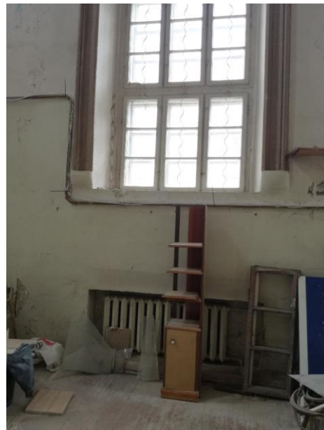
Figure C20: Radiator niche underneath the long window. (Author, 2018).
