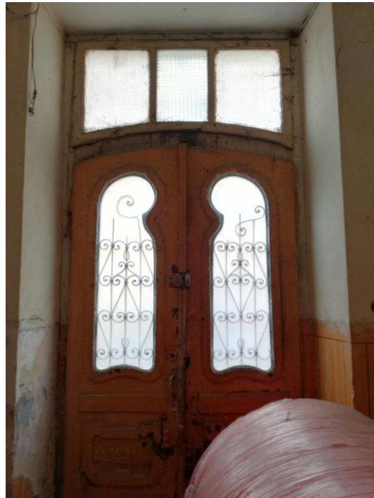
Figure C2: Main door. View from the inside. (Author, 2018).
