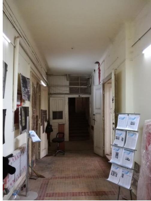
Figure 2-12: Hallway on the ground floor. (Author, 2018).
