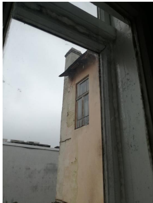
Figure C30: Staircase window. Third half-floor. (Author, 2018).
