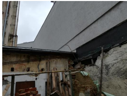
Figure C8: New building adjacent to the synagogue from the west. (Author, 2018).
