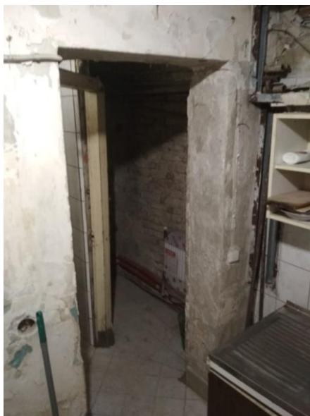
Figure 2-32: Toilets. Entrance to the toilet units. (Nazar, 2018).
