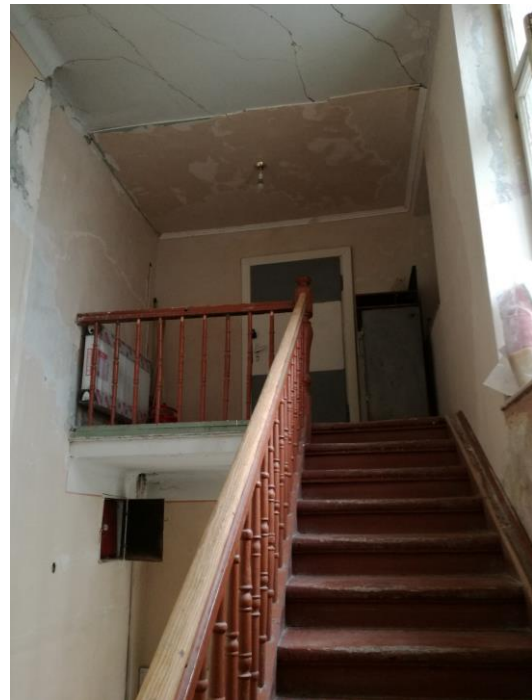
Figure 2-45: Staircase. Third floor. (Author, 2018).
