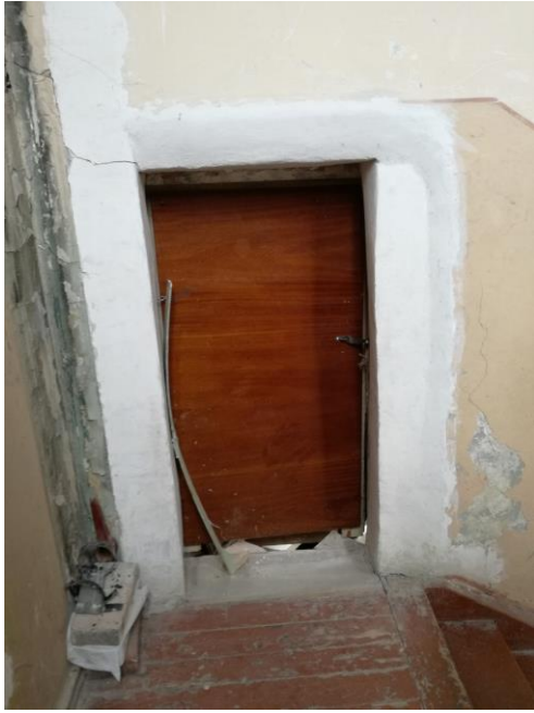
Figure 2-42: Staircase. Doors on the third half-floor. (Author, 2018).
