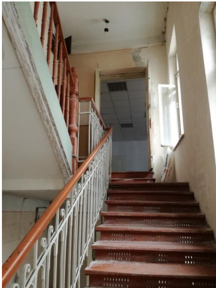
Figure 2-38: Staircase. Second floor. (Author, 2018).
