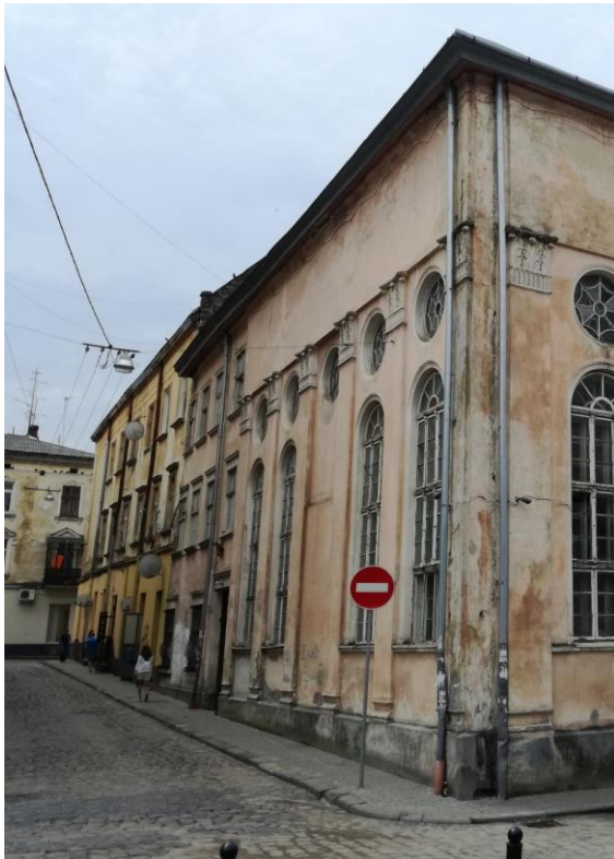
Figure 2-9: East facade. (Author, 2018).
