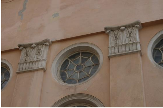
Figure C5: Pilaster detail. (Nazar, 2011).
