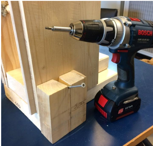
Figure 3-10: Attaching the Termowood element to the middle sill with a 60-degree angle screw connector.
