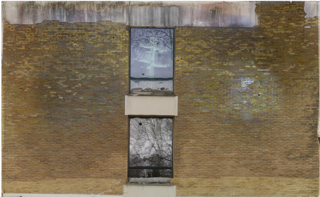
Figure 6.10: Orthophoto from a merged project with images from the camera attached to the Phantom 4 and also a Nikon D600 camera taken from the ground. The variation in white balance and light conditions are evident. One can see the difference in white balance of the top and bottom window. This effect comes from different light conditions during exposure, but also an unfortunate slip of poor image management, as photos with wrong white balance settings were added. Still, geometric distortions can be seen in the lower part of the orthophoto. Excluding that lowest part, the sharpness and detail was better after adding the terrestrial sourced images.
