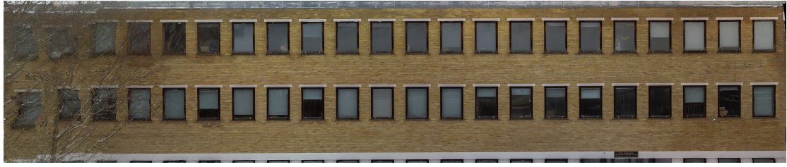
Figure 4.9: Orthophoto of KA-building, South wall.
