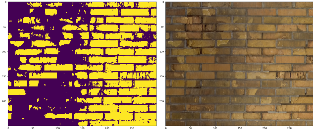
Figure 6.7: The success of the segmentation by the k-means algorithm varies across the orthophoto.
