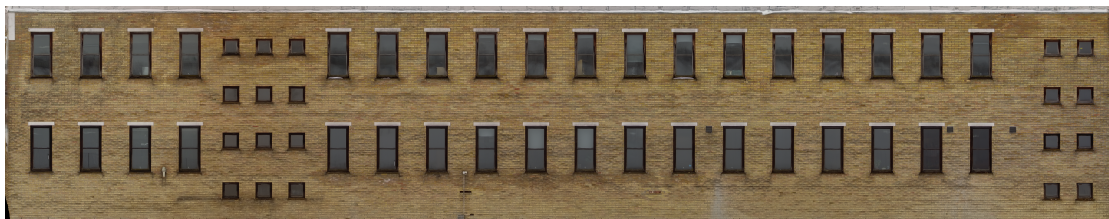
Figure 4.8: Orthophoto of KA-building, North wall.
