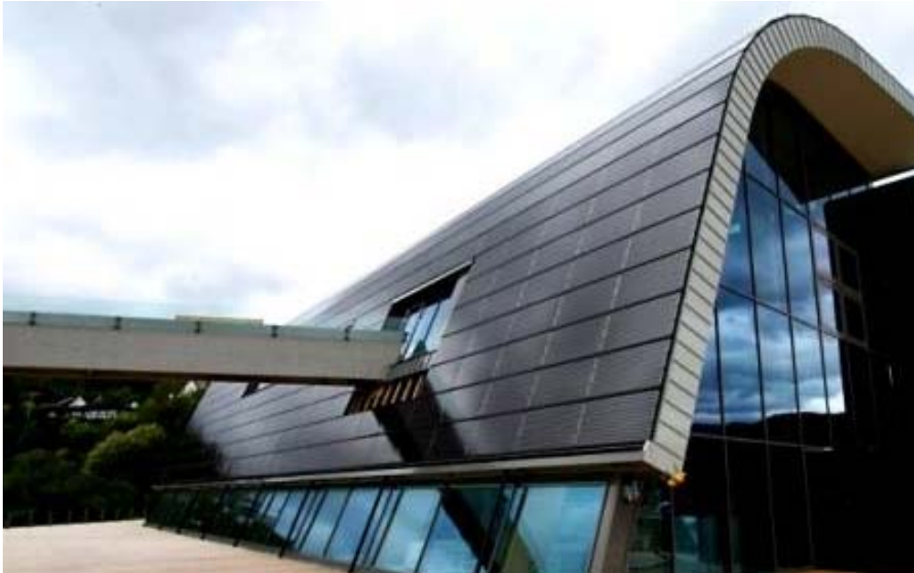
Figure 4-12 BIPV in façade. Source: Getek / fornybar.no
