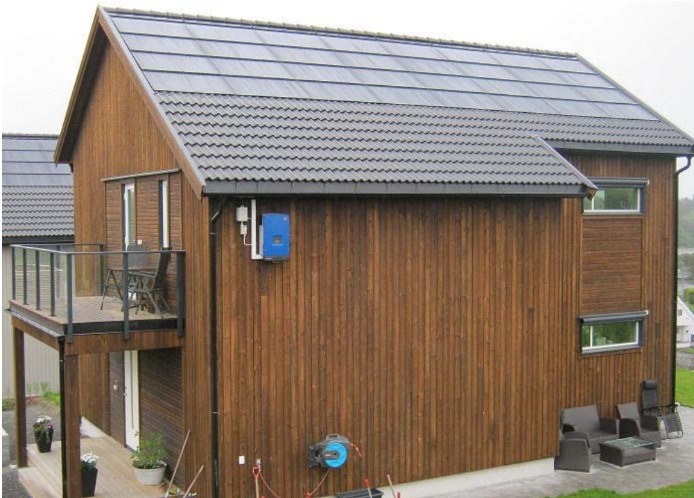
Figure 4-11 BIPV on a tilted roof. Source: bipvno.no
