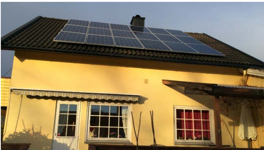
Figure 4-10 BAPV installed on the roof of a residence. Photo: Hege Westskog (Cicero.no)
