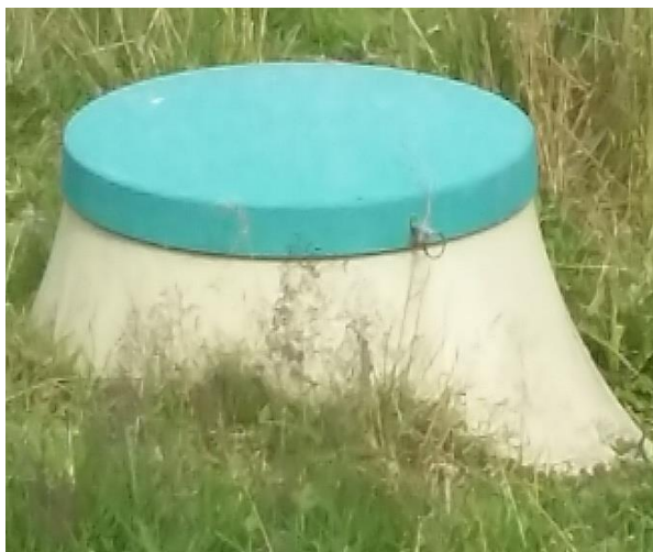
Figure 2: Fiber glass septic tank, having 4 m 3 volume and 3 chambers
