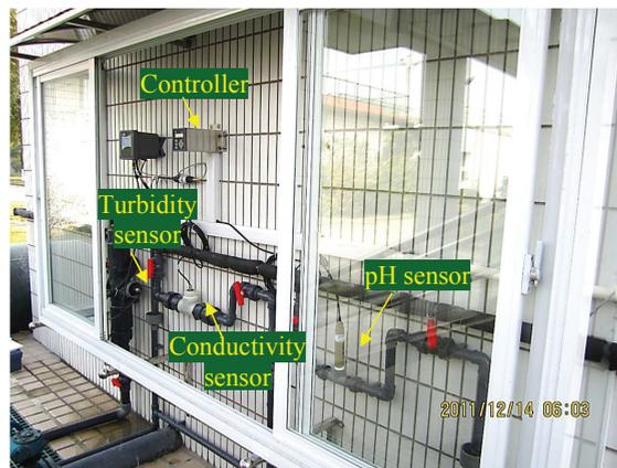
Figure 4. Inlet online instruments of N2DWTP. Including 3 inlet sensors: turbidity, conductivity, pH as well as sensor controllers
