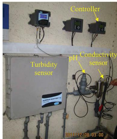
*Figure 7. Inlet online instruments of SDWTP. Three sensors are used for measuring turbidity, conductivity and pH*
