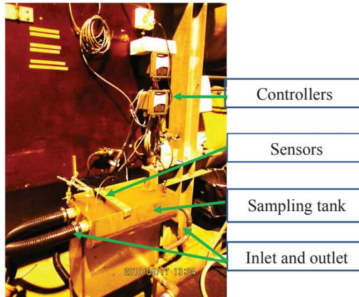
*Figure 9. Inlet online instruments of NRA WWTP. Three sensors measure turbidity, conductivity and pH*
