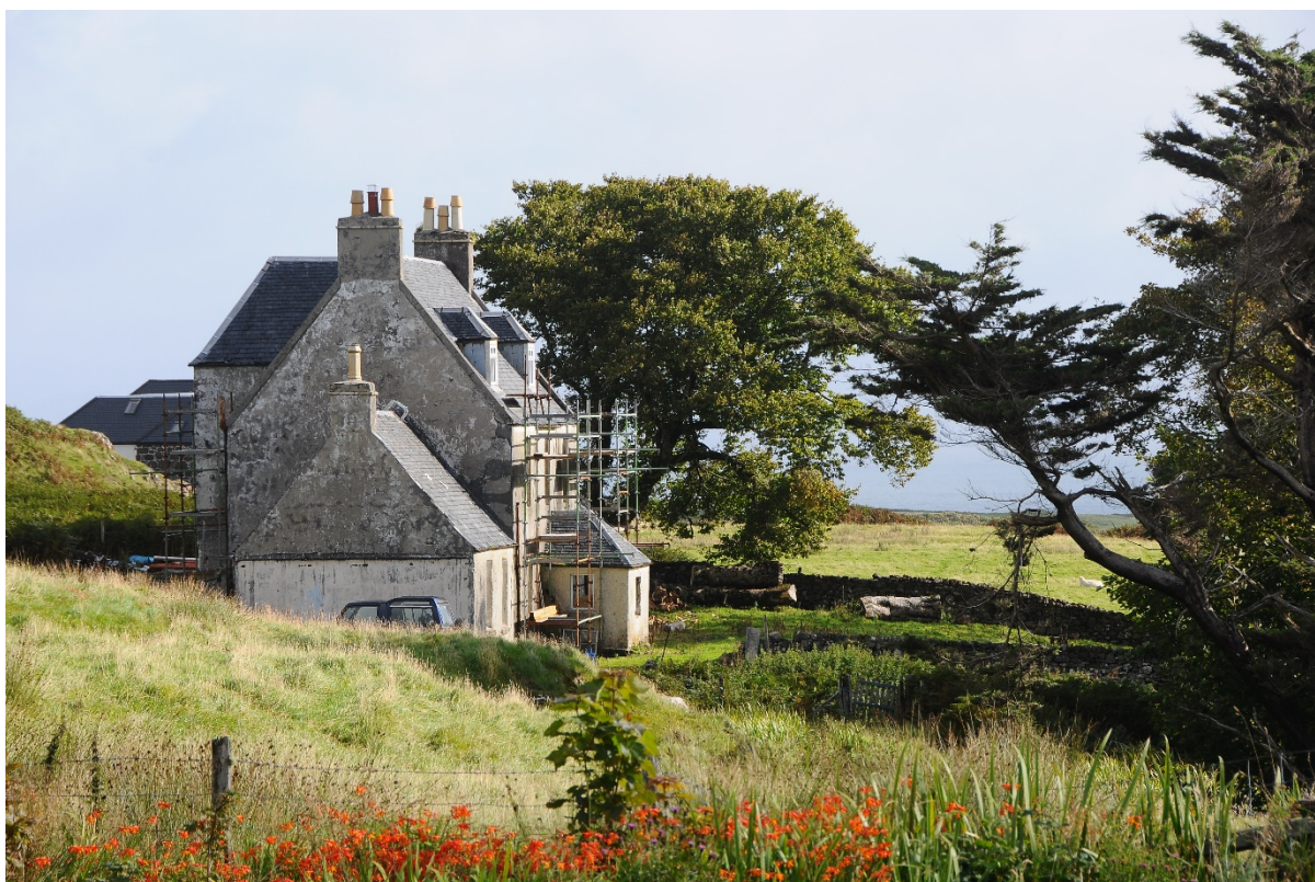
Figure 79 (Elic_085). The Manse under renovation.
