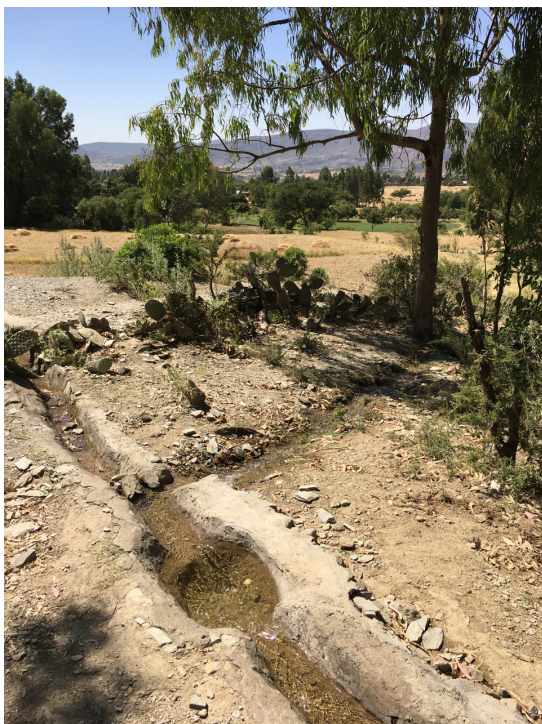
Image 5: The spillway that leads water from a spring down to the households in the Mountain Valley. Note the rudimentary water gate of stones that divert water to the shallow trench to the right.
