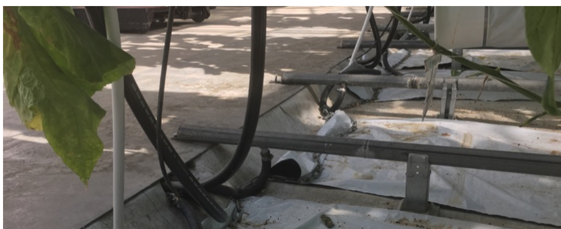
Figure 5-3 Step down from concrete floor is steep and provides no climb assistance. Also, the white plastic sheets seen between the rails are loose and slippery.
