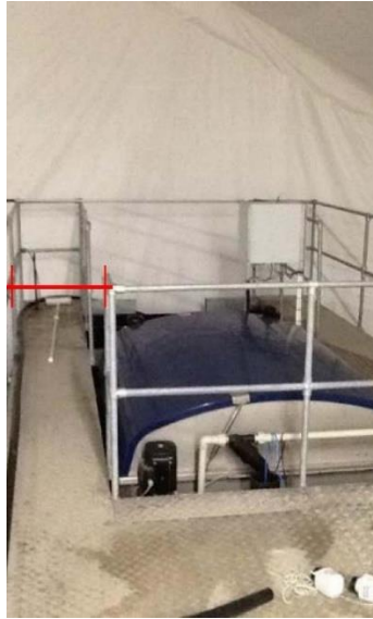
Figure 7.1.1: Footbridge with approx. 1 metre distance between railing
