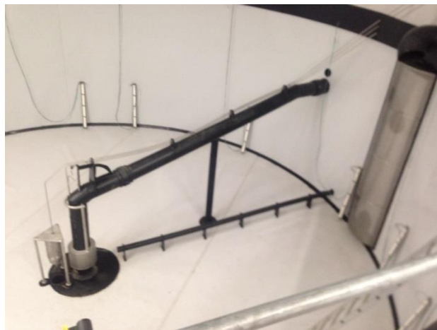
Figure 3.7.3.3: Dead fish collector transfer system (Levik, 2017b).
