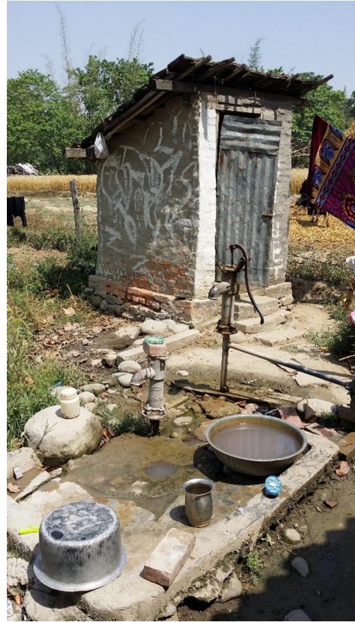
Figure 24: Pump well right next to toilet using pit (Photo: Anders Rørå)
