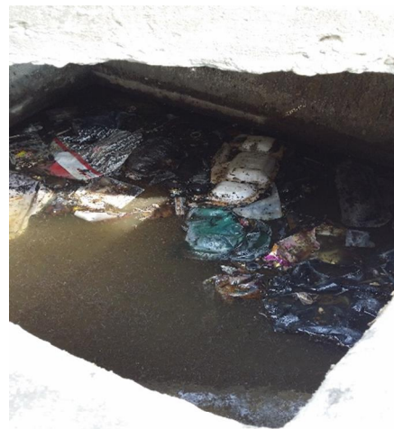
Figure 19: One of the septic tanks were filled with garbage and aquatic insects (Photo: Anders Rørå)
