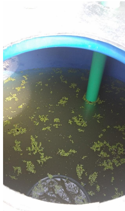
Figure 16: Duckweed in the pump tank (Photo: Anders Rørrå).
