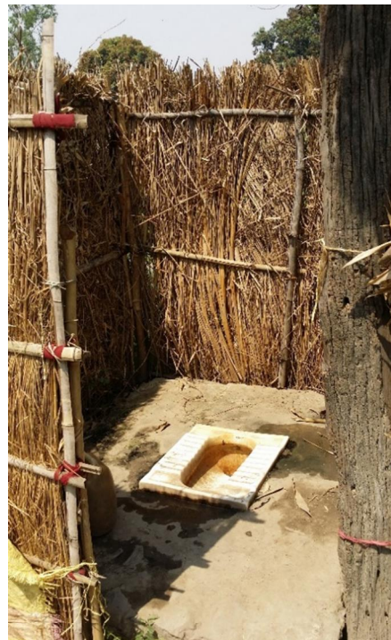
Figure 26: Toilet with superstructure built of straw (Photo: Anders Rørå).
