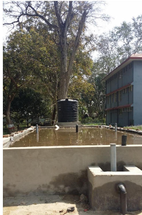
Figure 7: The whole system with biofilter in the plastic tank at the end and effluent from the CW in the pipe nearest in the picture. The water level was kept high the beginning to facilitate plant growth (Photo: Anders Rørå).
