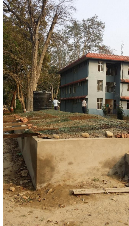
Figure 20: The constructed wetland had to be covered to protect the plants from being eaten by monkeys (Photo: Anders Rørå).
