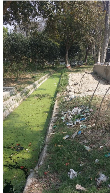
Figure 5: The effluent is discharged into this open drain (Photo Anders Rørå)
