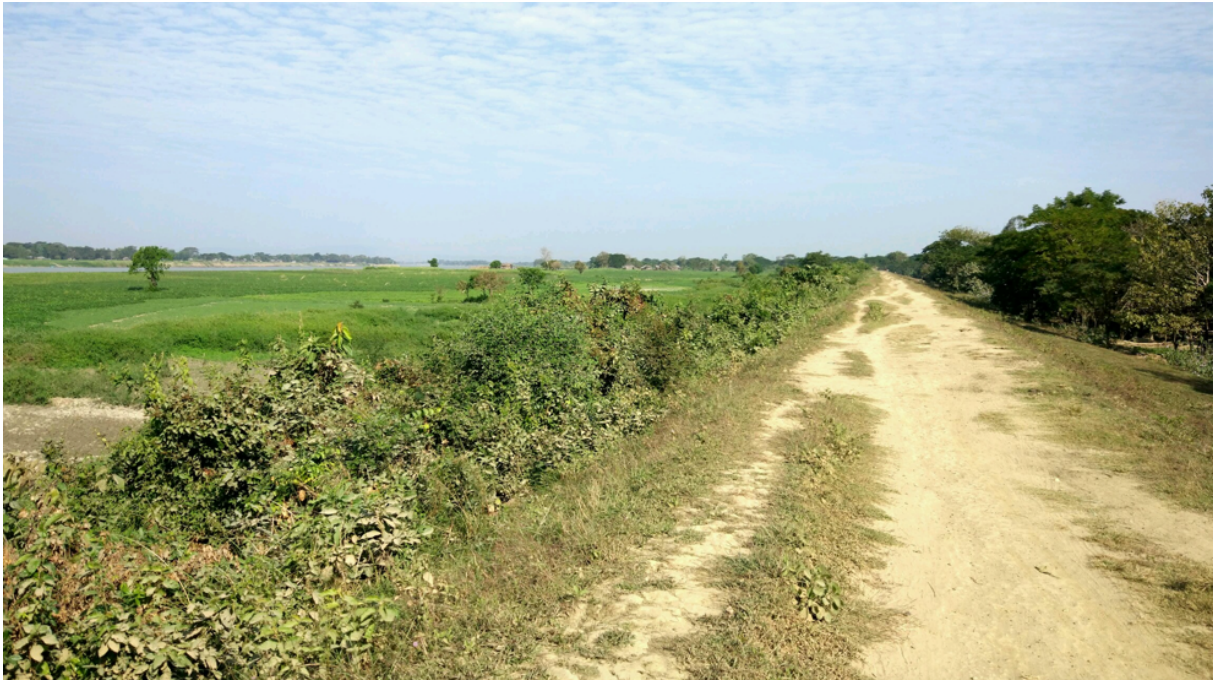
Photo 2: River embankment in Northeast Thabaung Township (Photo by Michael Foster, 2017)
