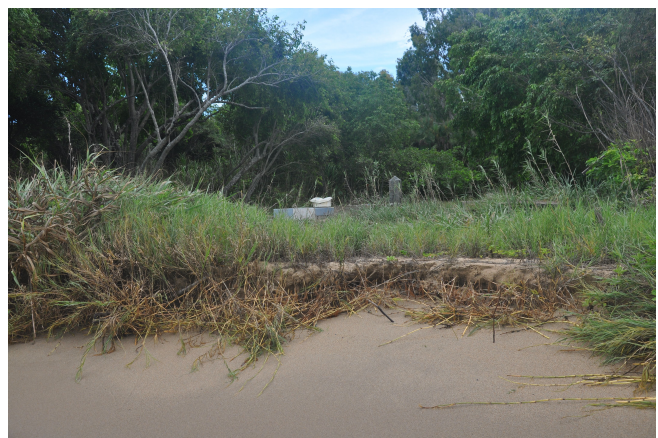
Fig. 5. Coastal erosion is encroaching on the cemetery of Monkey River village, Belize.
