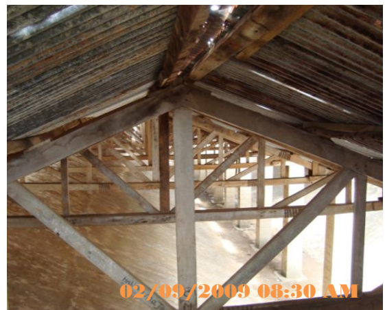
Figure 18: Empty water reservoir at Jibondo
