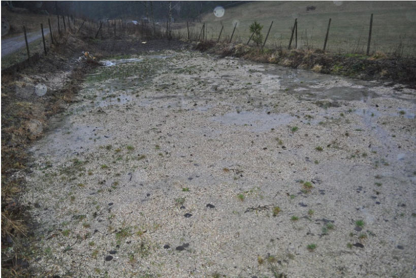
HF Constructed wetland
