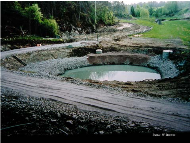
AFP during construction phase
