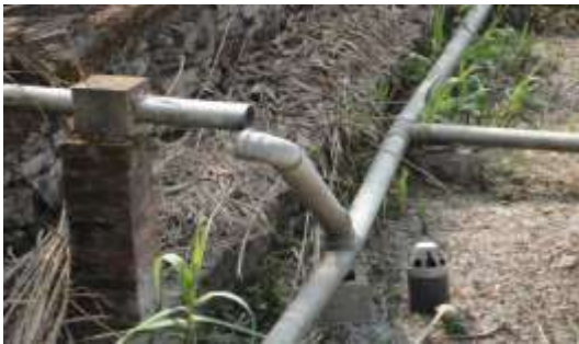
Disconnection of pipe from HFBs
