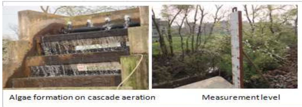
Figure 22: Field observation at Bhaktapur Jagati Treatment Plant
