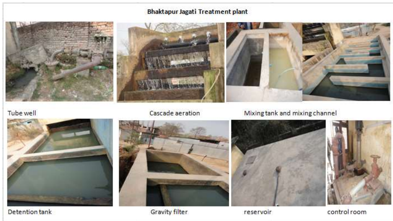
Figure 7: Pictorial representation of Bhaktapur Jagati Treatment Plant
