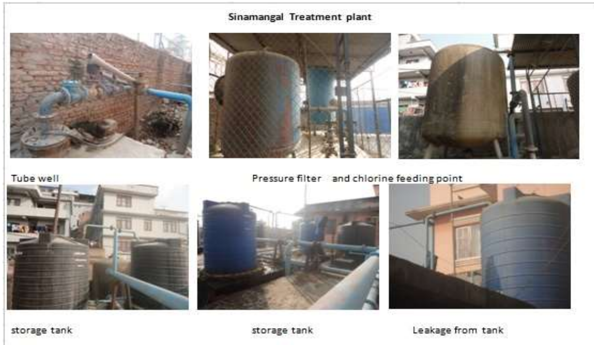
Figure 25: Observation at Sinamangal Treatment Plant
