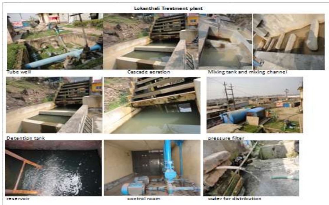
Figure 5: Pictorial representation of Lokanthali Treatment plant
