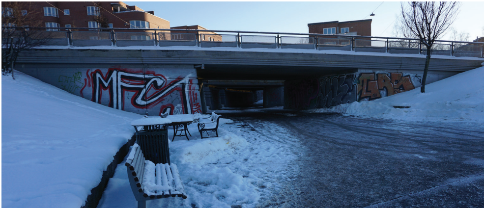
Figure 36. Picture delineates the tunnel, which serves as the entrance.
