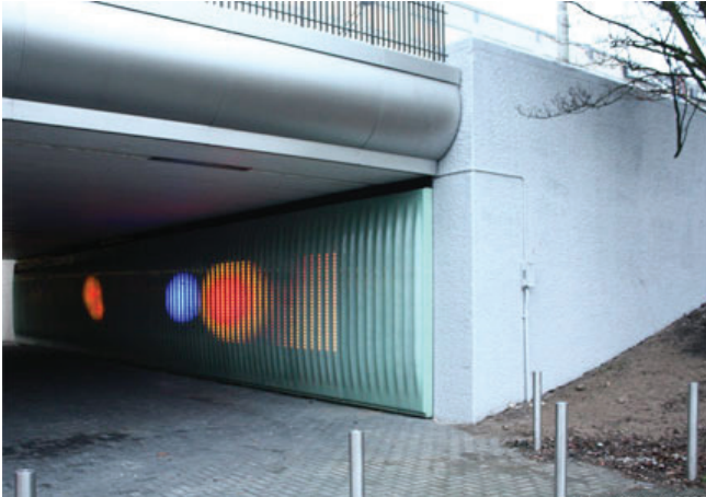
Figure 88. Inspiration: tunnel in Amsterdam.
