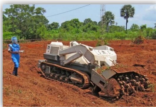
Figure 12: Digger D-3 with a tiller system [19].
