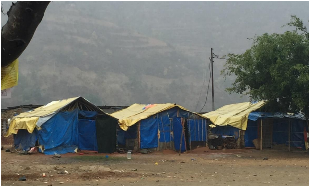
Photo 1: Temporary Houses in outskirts of Manthali Municipality
