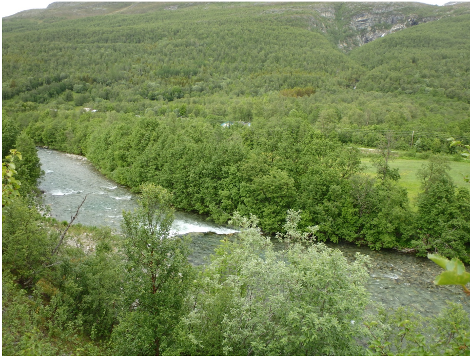
Figure 18. Picture showing weir and boulder structures in zone 7 in main river. The creek ravine of river Korselva can be seen in the background.
