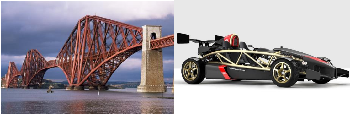
Figure 2-3. The Forth Railway bridge in Scotland and The Ariel Atom are both well known truss and space frame constructions and used in entirely different contexts [12] [13].
