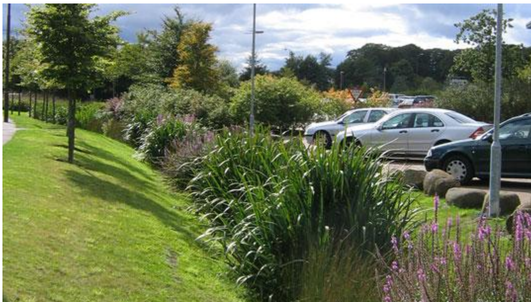
Figur 18: Dyp grøft gir god avledning av overvann, England. Kilde: http://www.local.gov.uk/suds-and-sabs/-/journal_content/56/10180/3578748/ARTICLE
