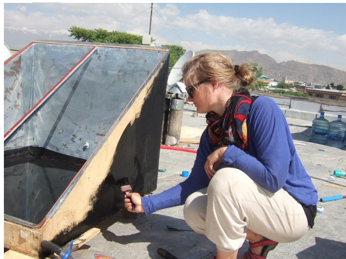
PICTURE 10: PAINTING THE PLYWOOD ON THE PLYWOOD SINGLE SLOPED SOLAR STILL
