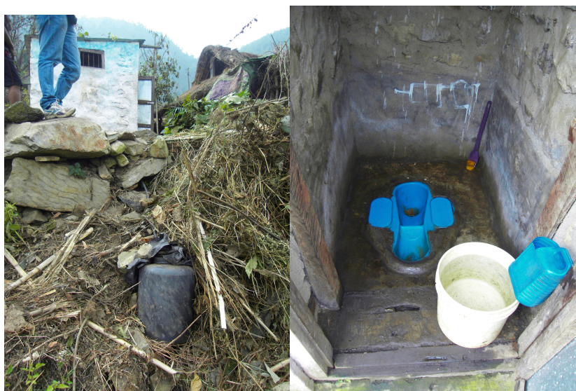
Figure 6: (photo: Kaia Bing) photos illustrating the eco-san toilets in Darechowk VDC.
