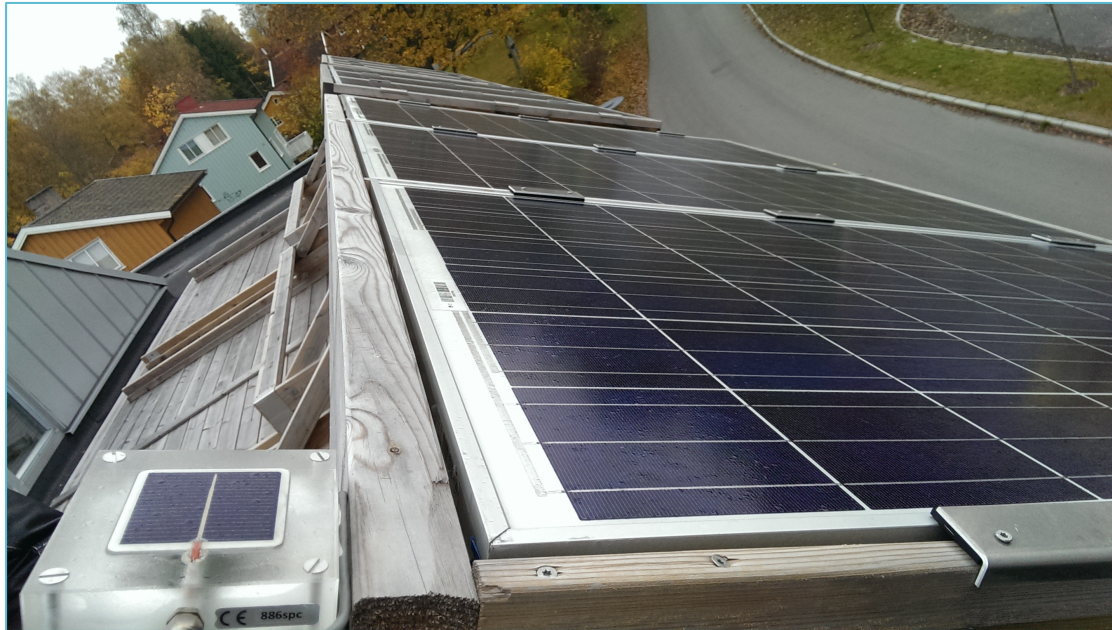
Figure 1: The PV-array at the campus of NULS at Aas, including solar reference cell
