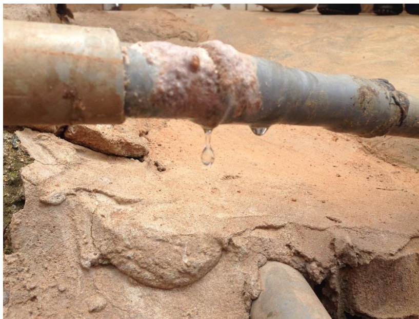
Leaking pipe
