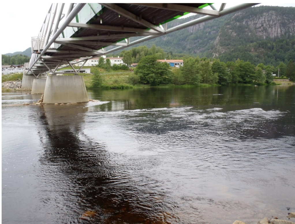
Figure 10. Station 3 (east bank - upstream direction).
