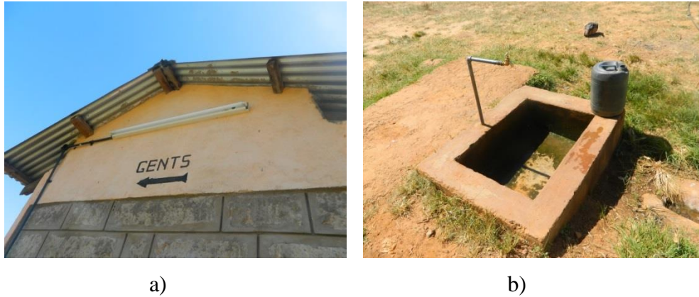
Figure 4.5. a) Lighting and b) hand washing facilities at the pit latrines at MCF Yatta. Photos: I. Georgiadis (2013).
