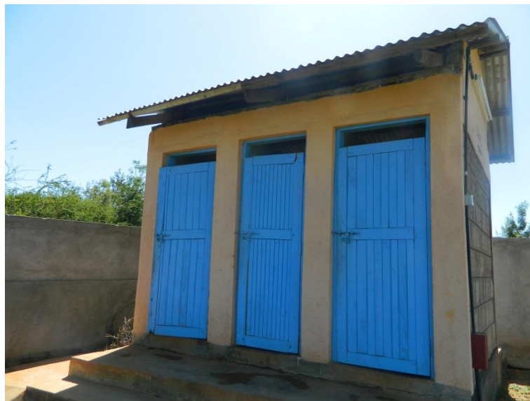
Figure 3.9. Pit latrines at MCF Yatta. Photo: I. Georgiadis (2013)
