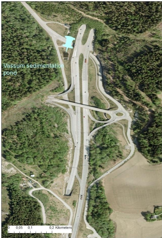
Figure 6. Orthophoto showing the E6 junction at Vassum and the sedimentation pond by the acceleration lane.
