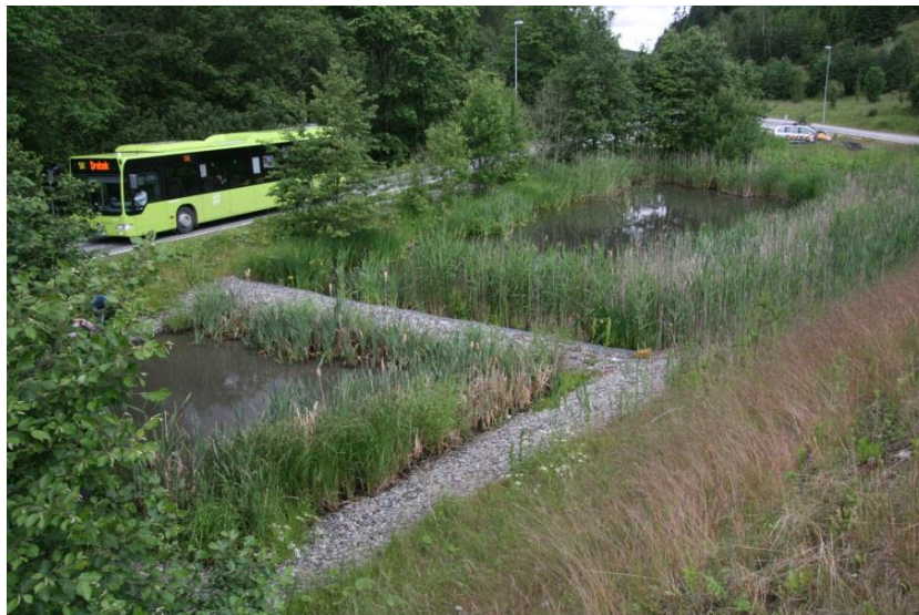
Figure 8. Vassum sedimentation pond seen from the inlet. Photo: Susanne Lund Johansen.
