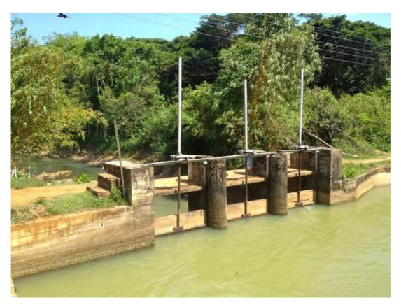
Figure 19 - Sluices that easily can be opened with a simple tool
