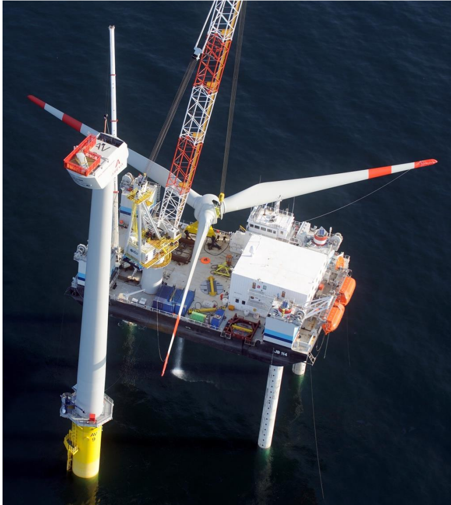
Figure 69: Installation of a preassembled rotor at Alpha Ventus (Wilmert 2013)
