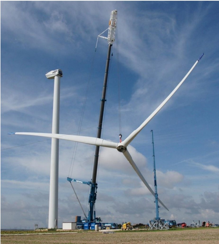
Figure 97: Installation of onshore wind turbine (Sarens Group 2013)
