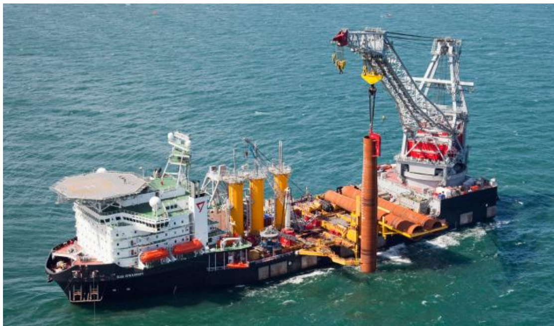
Figure 37: Shows Oleg Strashnov installing monopiles (Gusto MSC 2012)
