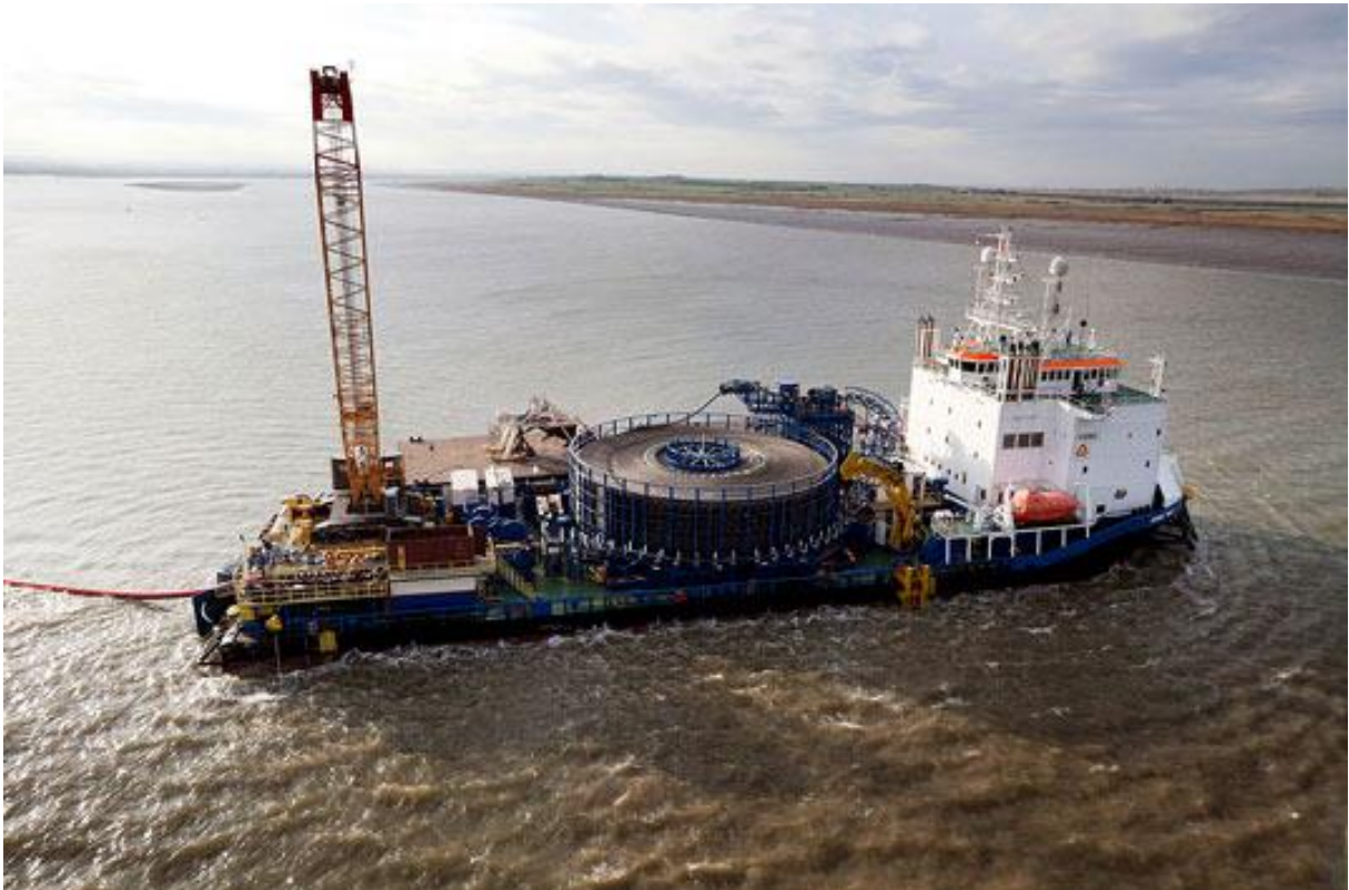
Figure 79: Cable installation by Stemat Spirit at London Array (London Array 2013)
