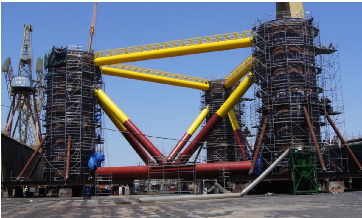
Appendix Figure 1: Manufacturing of the WindFloat pilot substructure
