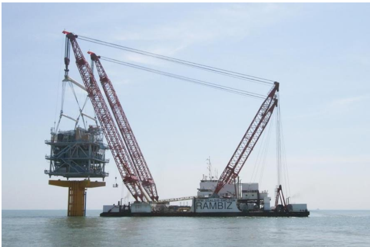
Figure 80: Offshore substation installation by Rambiz at London Array (Mercator Media 2013)
