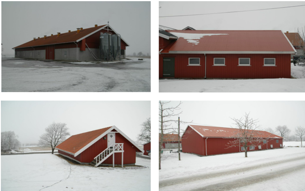
Figure 35: Southward-facing roofs on the chicken house(upper left), the grain storage building(upper left), the garage(lower left) and the vegetable storage building.
