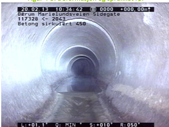
Figur 4-5: Svank 1 meter frem
