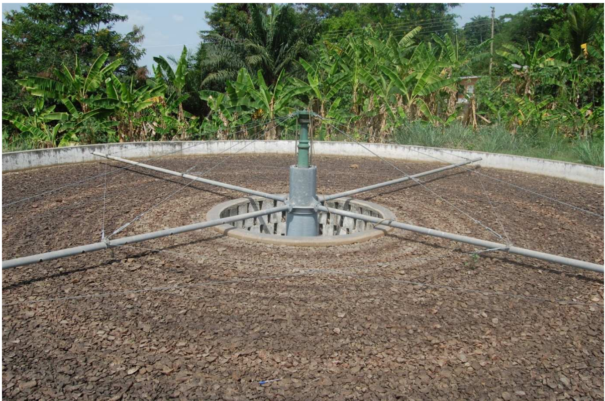
Figure 9: Trickling filter
