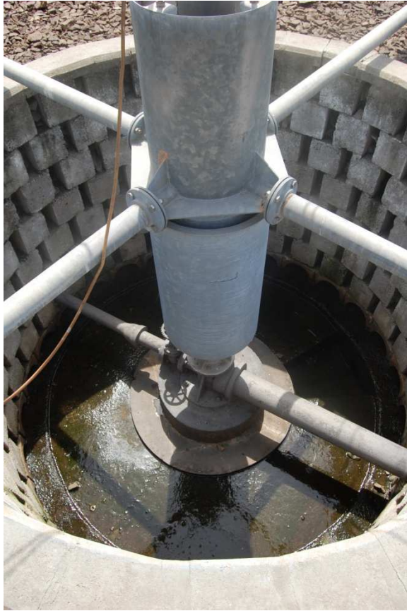
Figure 10: Pivot of trickling filter
