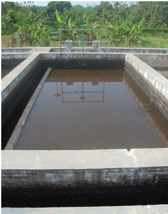
Figure 14: Filled tertiary treatment basin
