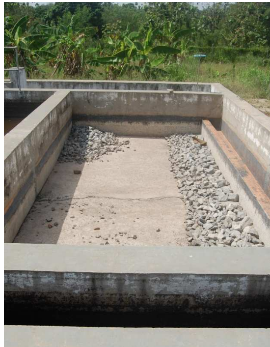
Figure 15: Empty tertiary treatment basin
