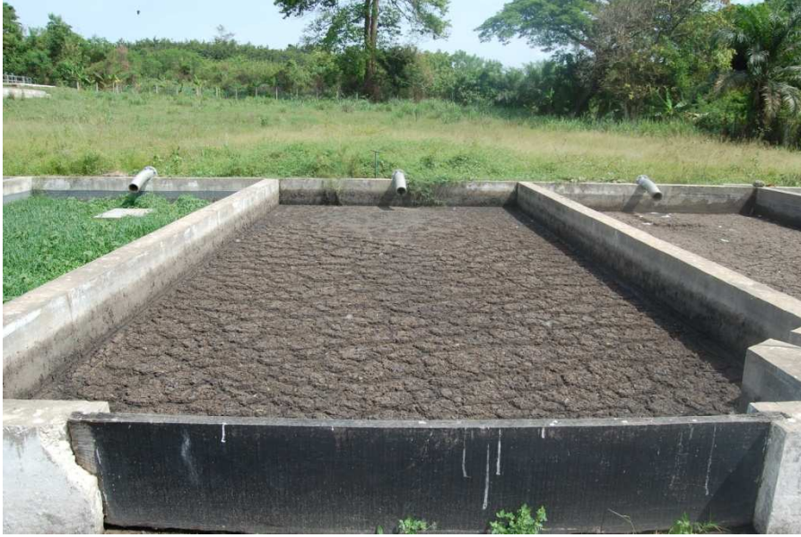
Figure 17: Single sludge drying bed
