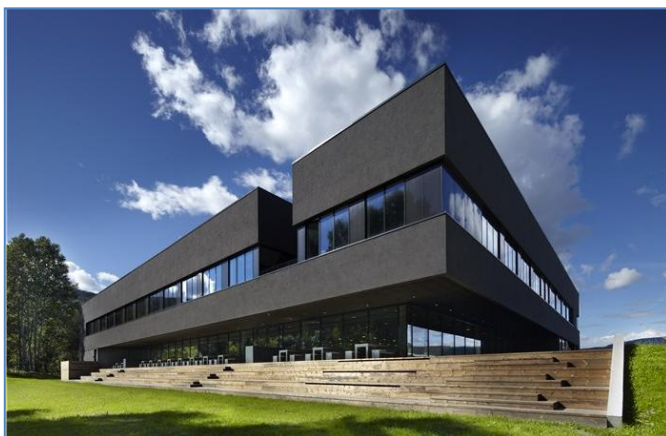
Figur 74 Marienlyst skole [futurebuilt.no]
