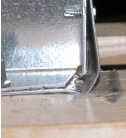
Figure 9: Buckling in the sheeting metal and compression of GLT. The picture is taken from Furulund and Thorrud's thesis.
