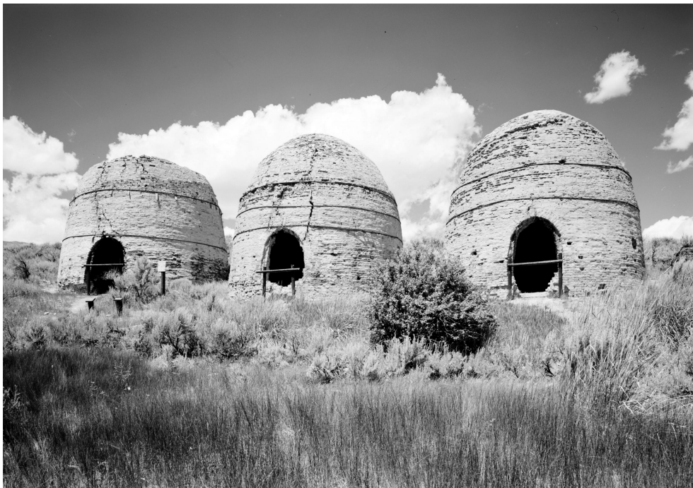
Figure 3.2: Picture of a Beehive charcoal kiln, located near Leadore, Idaho, USA. Photo: James A. McDonald. Public domain[19].
