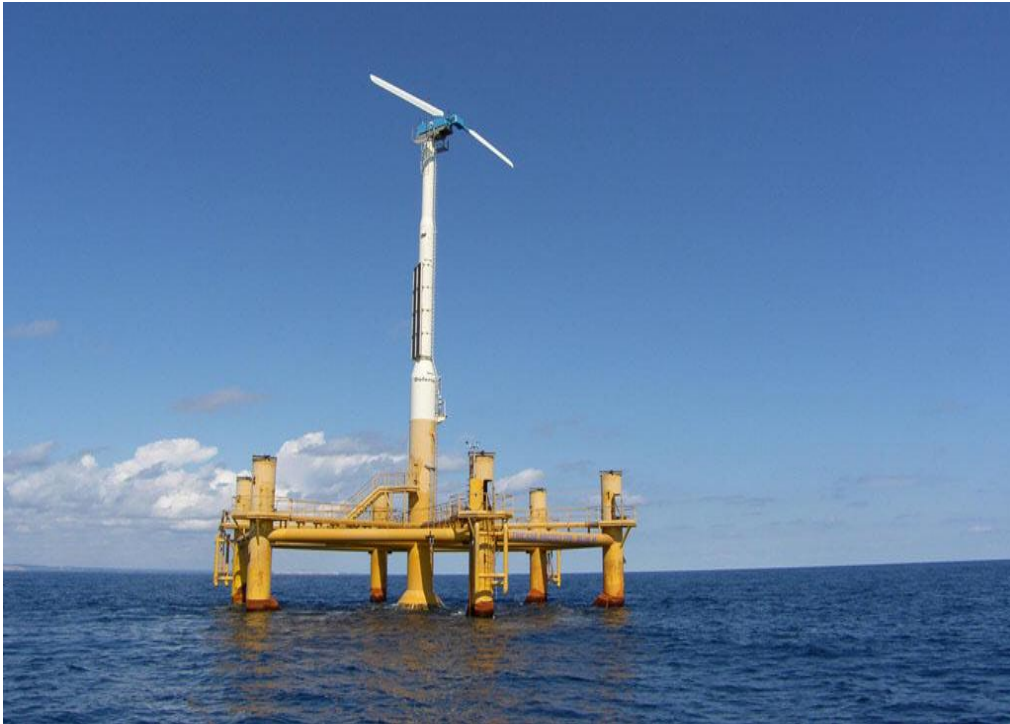
Figur 14 Blue H under testing i Middelhavet, (Blue H Group, 2010).
