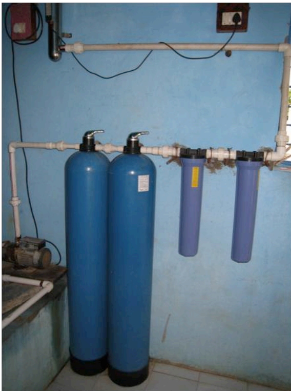
Picture 14 and 15: Upputuru, sand filter followed by a activated carbon filter, 10 micron bag filter, 5 micron bag filter and a UV unit (left upper corner) (left). Reject water handling (right) (Havig and Holstad, 2010).
