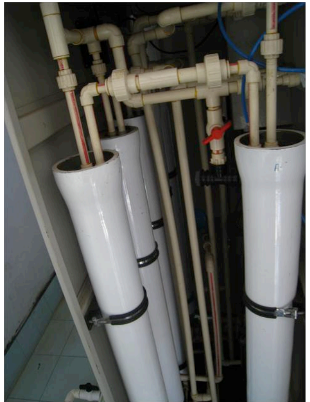
Picture 18 and 19: Remalli, dual media filter followed by activated carbon filter (left), and the membrane filter modules (right) (Havig and Holstad, 2010).
