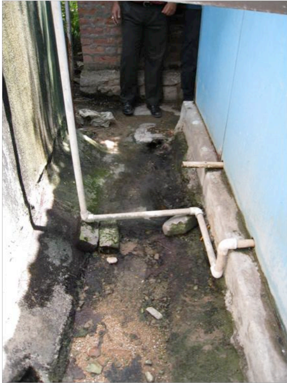
Picture 24: Katcharam, the plants raw water intake (nearest pipe), and the reject water expiry (Havig and Holstad, 2010).
