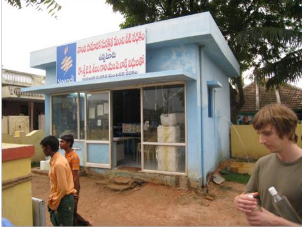
Picture 13: Upputuru, the drinking water purification plant (Havig and Holstad, 2010).
