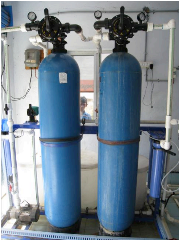
Picture 18 and 19: Remalli, dual media filter followed by activated carbon filter (left), and the membrane filter modules (right) (Havig and Holstad, 2010).
