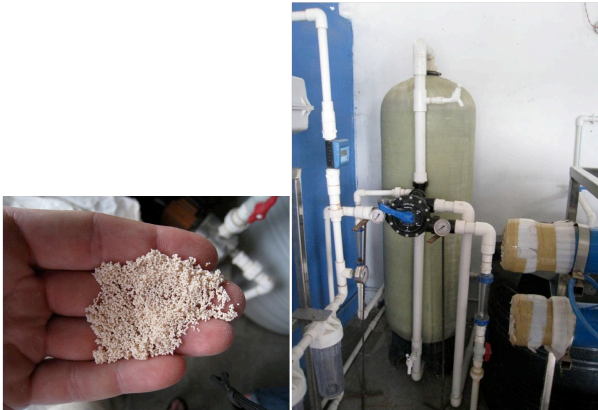
Picture 5 and 6: To the left is used activated alumina. The right picture shows a column filter filled with alumina. Both picture are taken at Devarapalli, Andhra Pradesh, India (Havig and Holstad, 2010).
