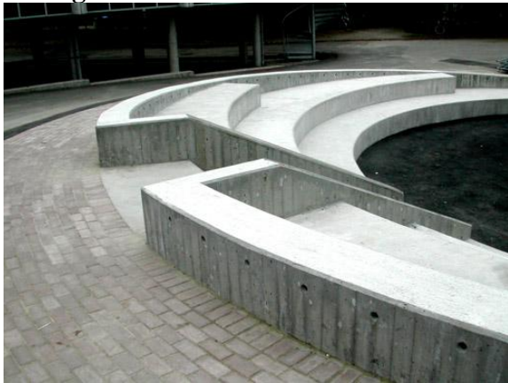
Foto 2: Betong. (SV Betong)
