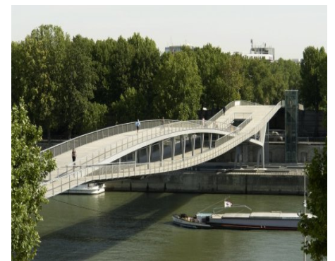
Figur nr. 18 Pedestrian Bridge Simone de Beauvoir
