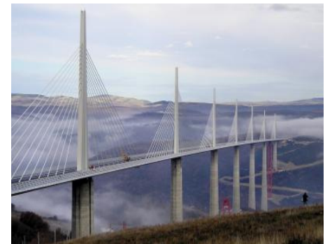
Figur nr. 17 The Millau Viaduct road bridge
