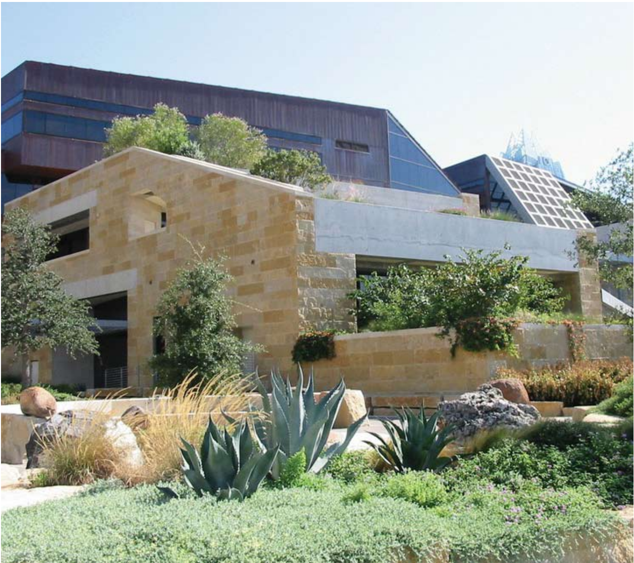
Figur 25b: City Hall i Austin, Texas. Foto: American Hydrotech (Green Roofs for Healthy Cities 2009a).
