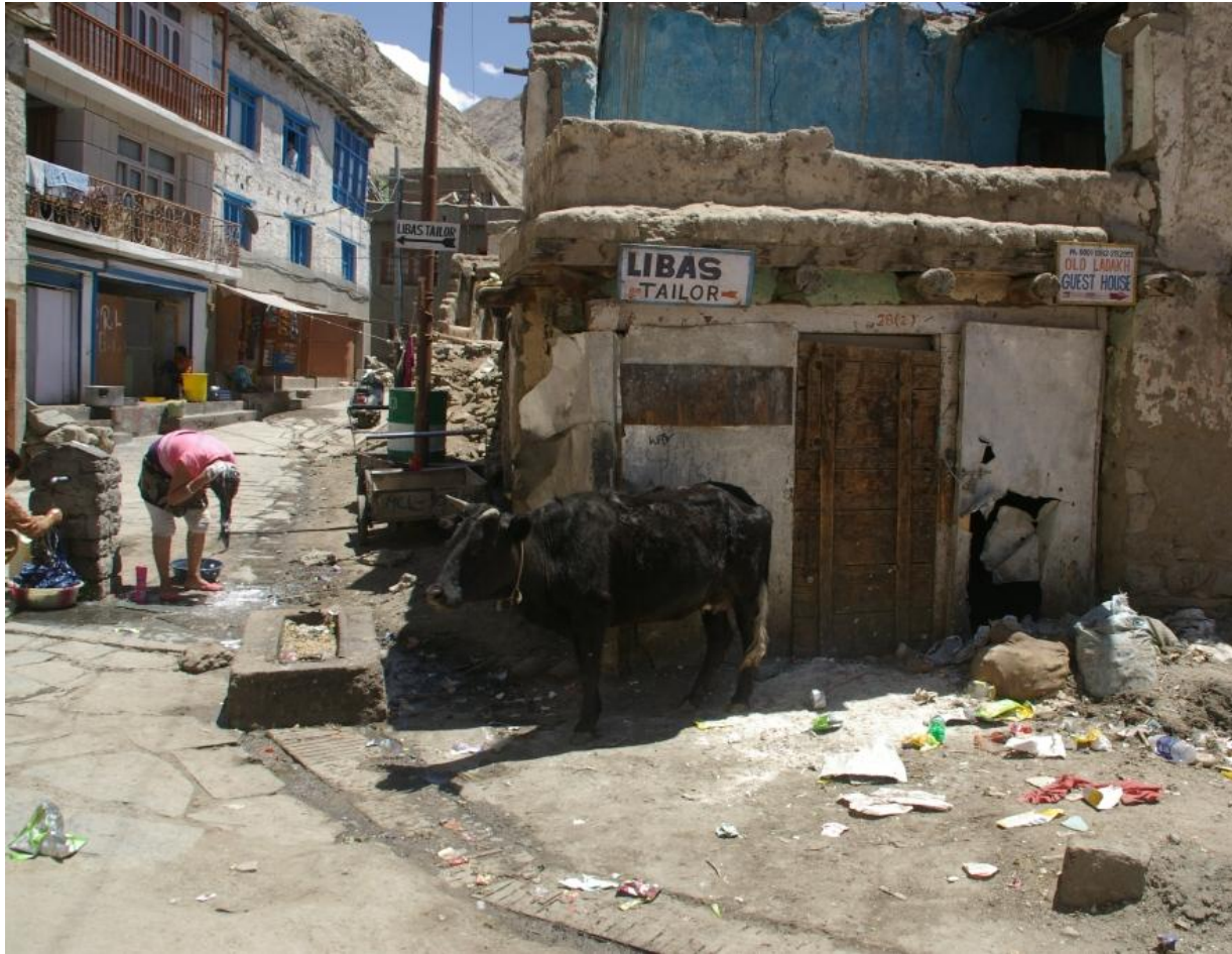
Figure 19 Area around the common water tap in Maney Khang where people are taking drinking water, washing clothes and hair. The office of the informant below is located just in front of this area and others also pointed out the untidiness of
