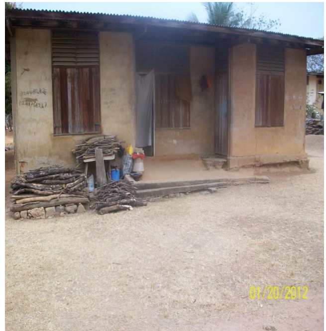
b. Resettlement house quite in shape
