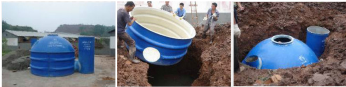
Fig.4. The pictures of GPR digester
