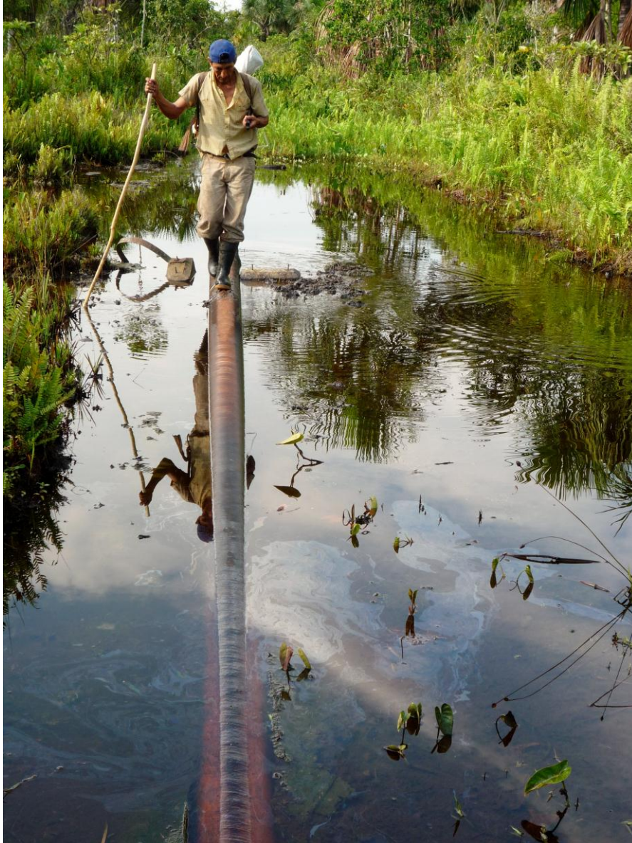
Figure 2. Forty-year old leaking pipelines in Pluspetrol's oil block 8E
