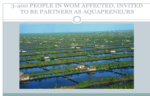
Photo 3: Aerial view of the aqua city in Indonesia
