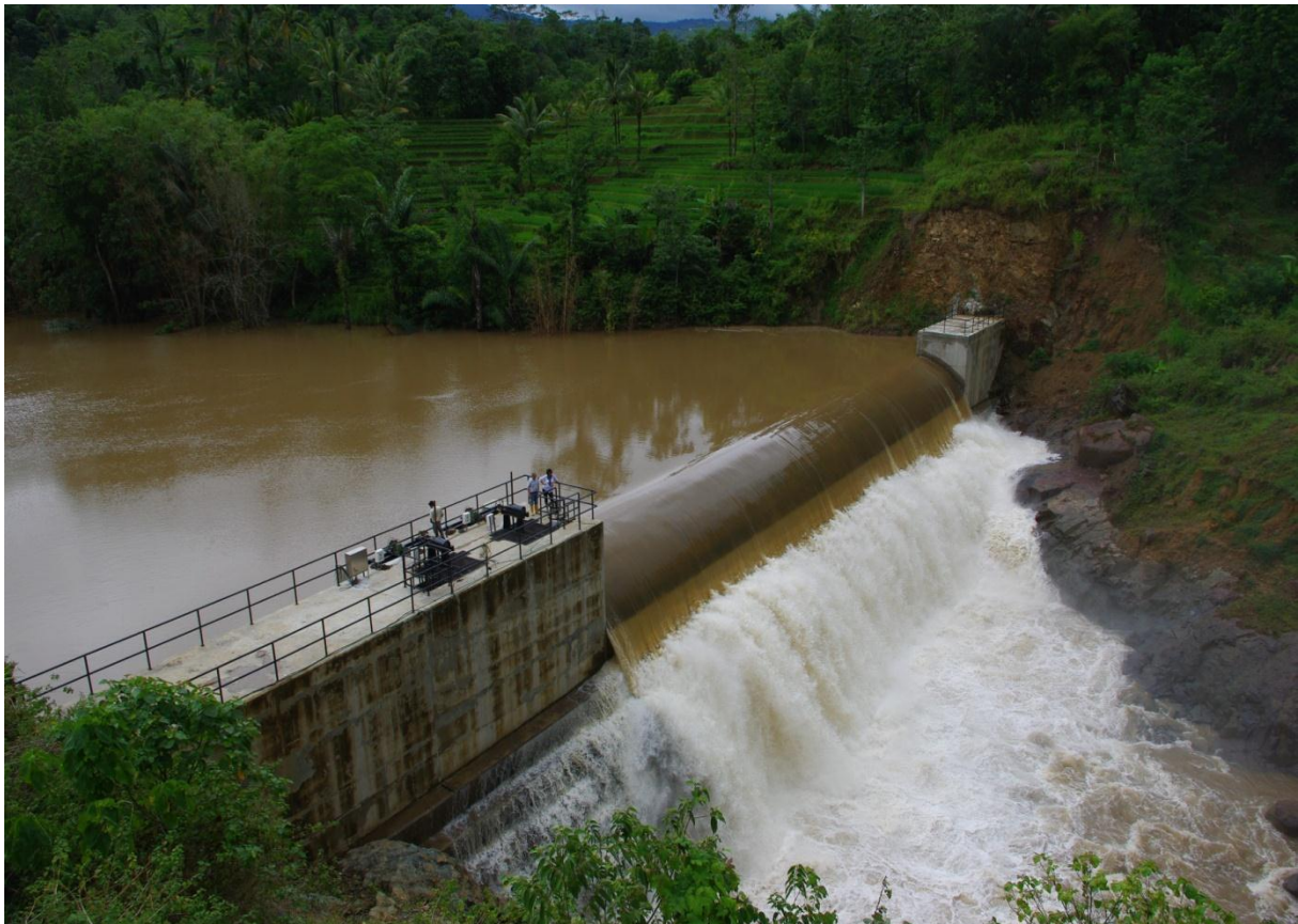
Manipi HEPP, 10 MW Hydro power project, Sinjai region, South Sulawesi, Indonesia
