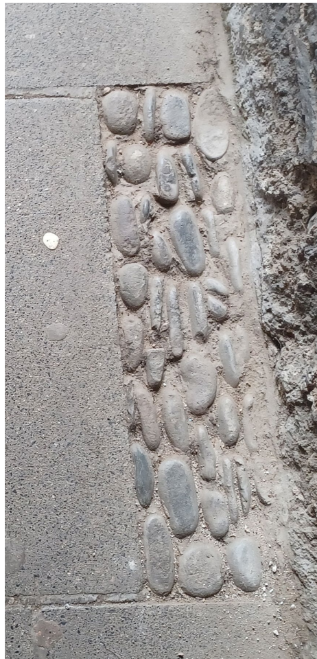
(Above) FIGURE 55: Pebbles are used to fill the gap in the pavers, Photograph by Molly Andrews
