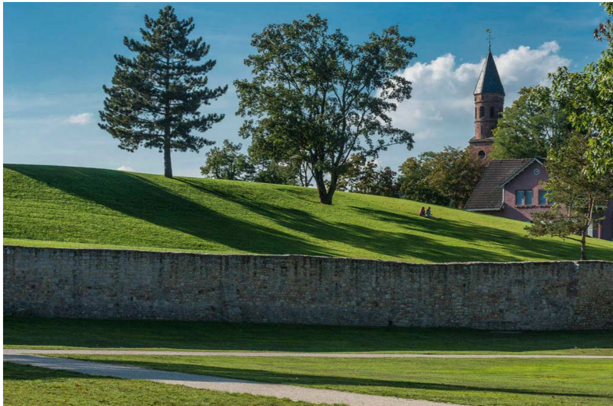
FIGURE 22: Example of 'the beautiful' UNESCO World Heritage Site Abbey Lorsch, by hg merz Architekten and Topotek 1 (Image source: Joosten, 2021)
