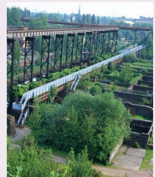
FIGURE 82: Walled gardens and promenade at Duisburg Nord (Landezine, 2011)
