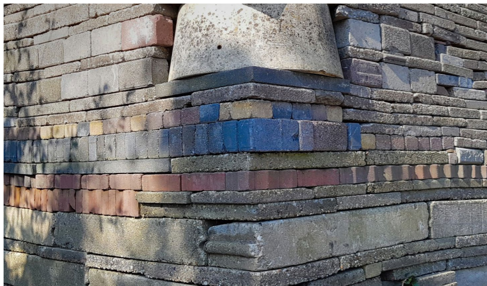
FIGURE 53: Detail of the stacking methods used at the Eco-cathedral Heerenveen. (Eco-kathedraal, 2021)
