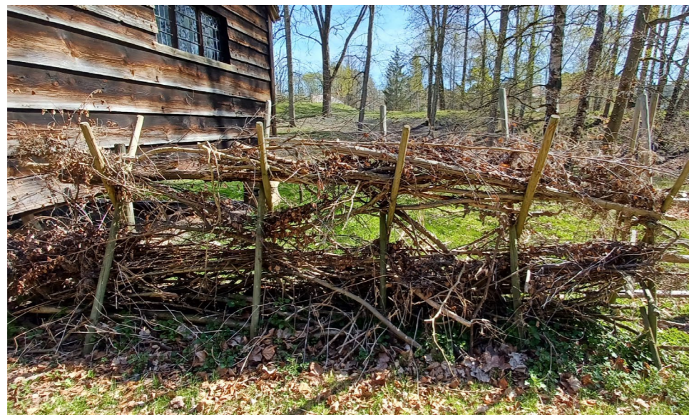
FIGURE 45: Fence constructed by a timber frame layered with cut branches to create a barrier (Photograph by Molly Andrews)
