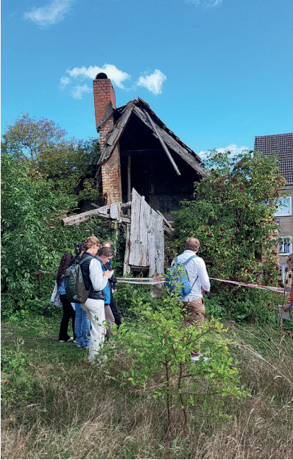
Half timbered wall construction with infill of clay and straw chaff. Photo: Terje Qvive
