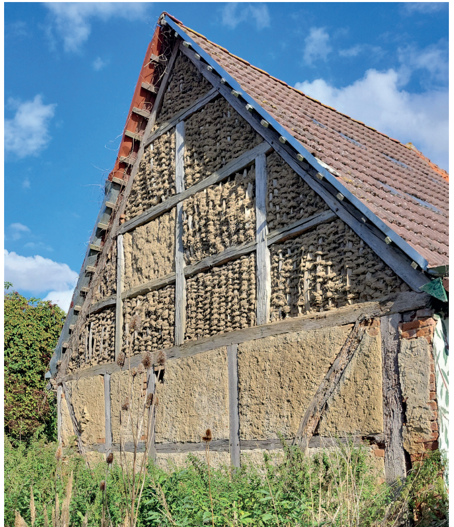
Half timbered wall construction with infill of clay and straw chaff. Photo: Terje Qvive
