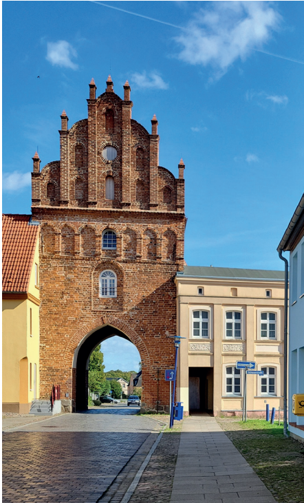
Two town gates dating to the 14th century: Mühlentor to the West and Steintor to the East. Both gates were recently repaired. Photos: Terje Qvive
